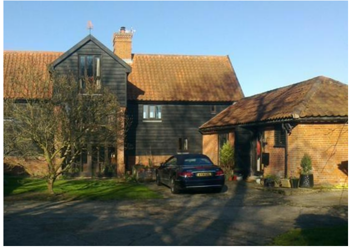
Above: Reydon Barn Conversion with weatherboarding Below: Older Reydon House with Colour Wash
